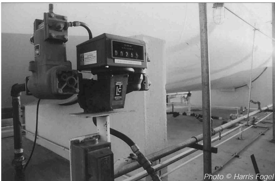
24-2 Meter/dispenser next to 30,000 gallon storage tank.
