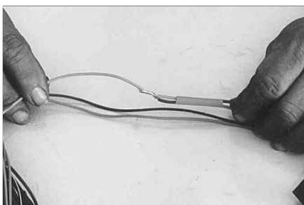
Step 4: Slip heat shrink over spliced OEM and tap wires, twist together all three wires – position heat shrink well away from solder joint.
