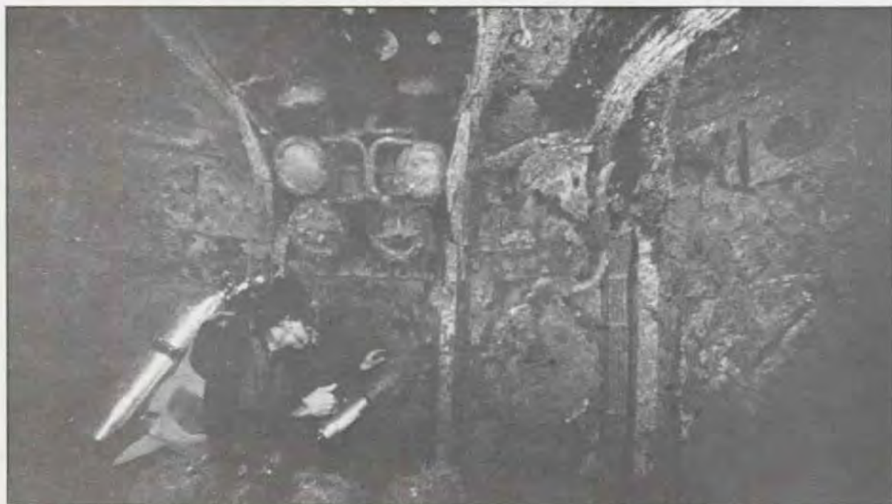
Catherine Courtney inspects the blast covers on Saratoga's bridge. (NPS, Larry Murphy)
