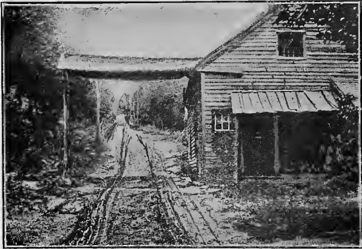
Old Toll Gate, Entrance to Clove Road.
