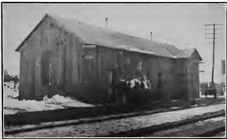
Temporary Depot at Catskill, built in two days after the destruction of the old depot at West Shore Station. View of first depot will be found elsewhere in book.
