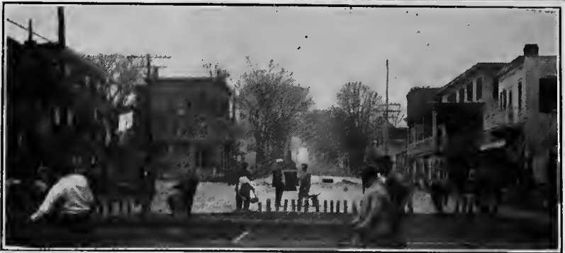
Laying Brick Pavement, West Bridge Street.
