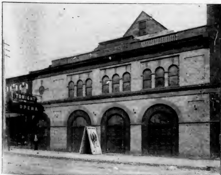
The above is a good reproduction of the Huntingdon Opera House at Huntingdon, Pa. The auditorium is on the ground floor and the balcony is on the main line of the Pennsylvania Railroad between Harrisburg and Johnstown. It draws from several small cities within
