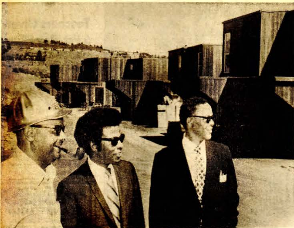
Bob Jackson, job superintendent, Eldridge Johns, manager of Trans-Bay Engineers, and Ray Dones, of the General and Specialty Contractors' Association, at new Navy hospital housing.
