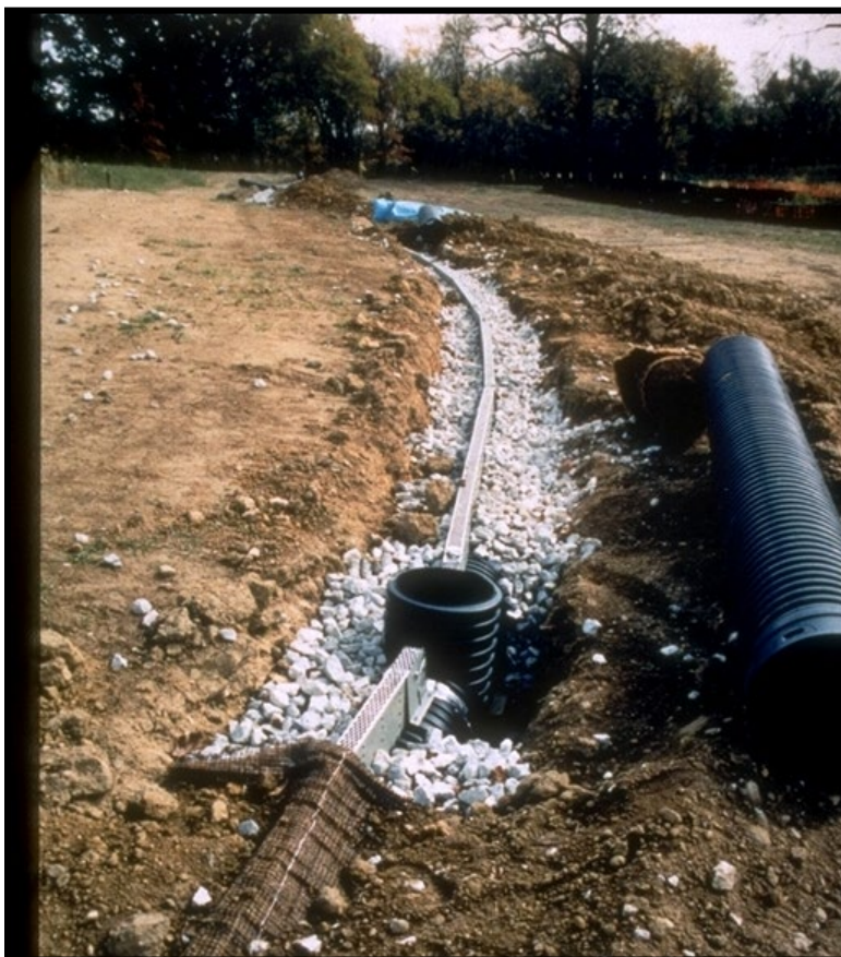
Figure E.7. Level Spreader Prior to Backfill and Downstream Stabilization.
